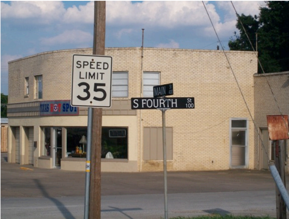
Home of Texas Hot Spot and Wallis Welding – 316 Main Street Garland Texas—located on the other side of the tracks. This interesting building, once home to an automobile dealership is currently repurposed into two businesses: 1) a retail nonprofit shop that sells liquidated merchandise to benefit a girls home in India and 2) a regionally acclaimed welding shop.
