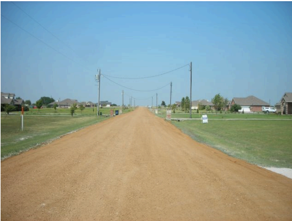
Example of Crushed Granite Road
