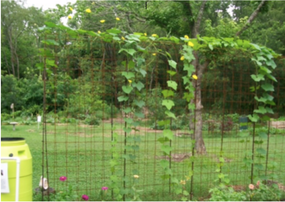
Charlie single handedly built the loofah tunnel in the spring of 2015. It is one of the outstanding features of the Garland Community Garden.
